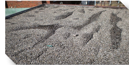
Gravel from tops of buildings
